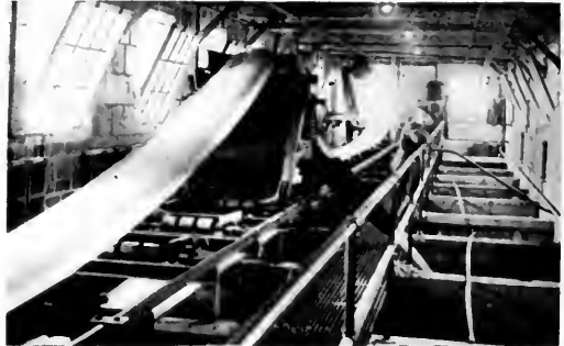
Chip Conveyor Belt, Tripper and Bins.
